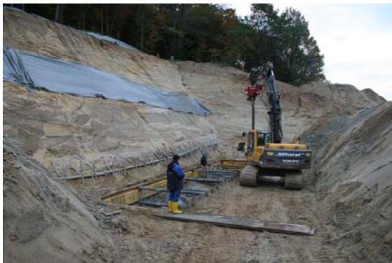
Quellbaugrube in Molassesanden
